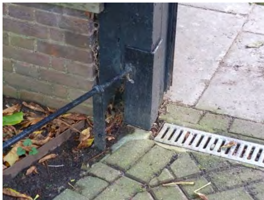
Rotten oak post adjacent to drainage channels (2.20). Steel reinforcement bolted to brickwork(2.21)
