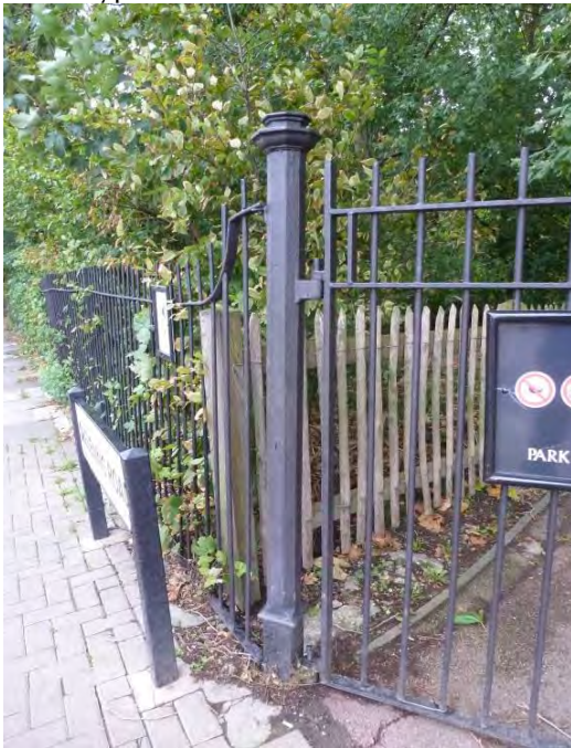
Cast iron gatepost
