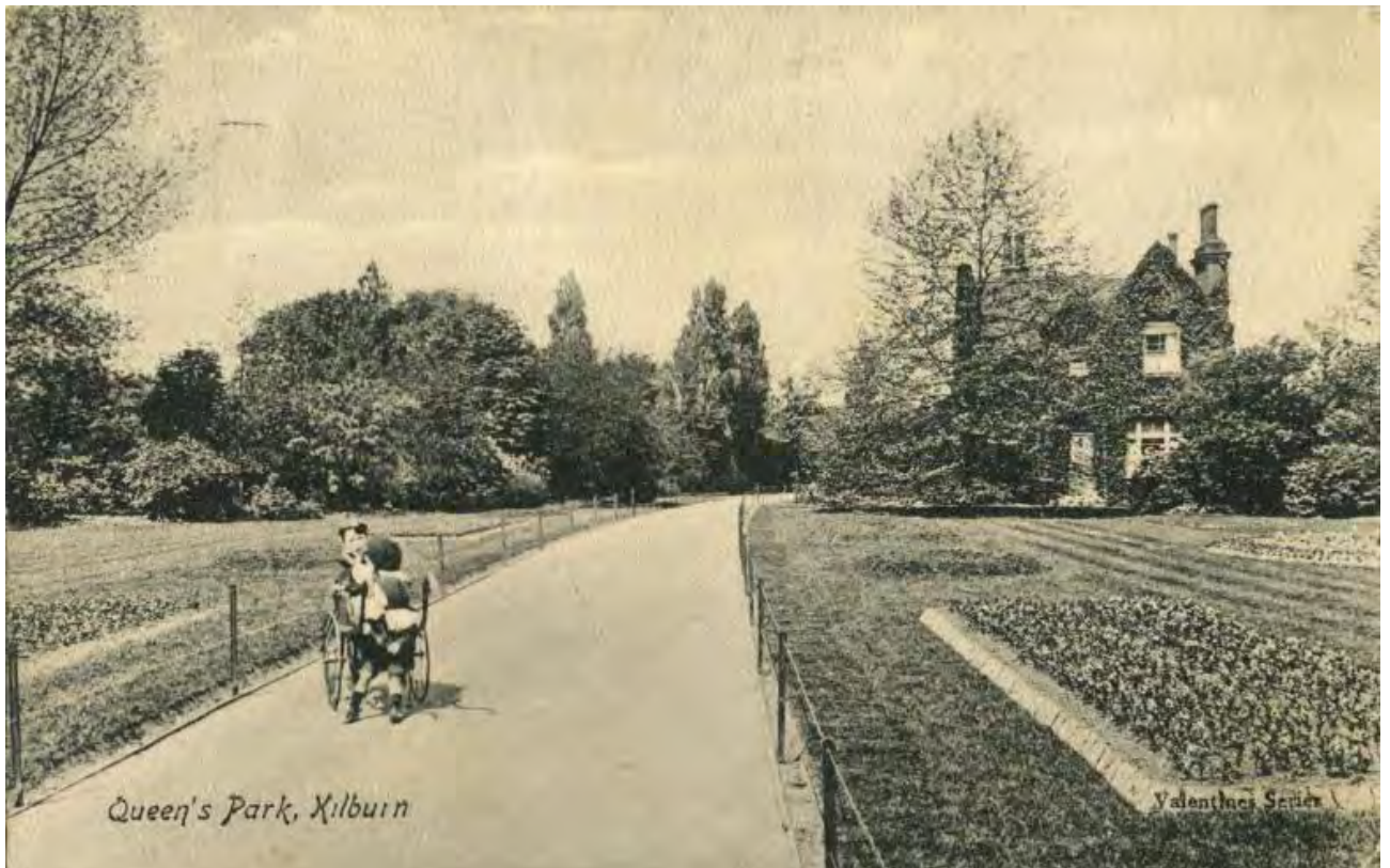
Figure 31: Postcard from 1900s showing lodge and post / wire fencing
