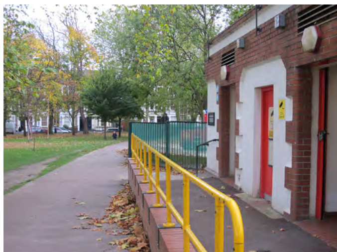
View south of toilet block
