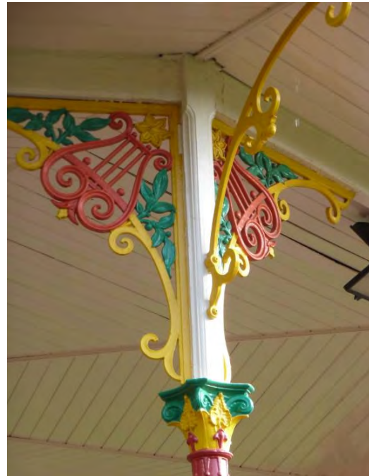
Detail of column bracketry
